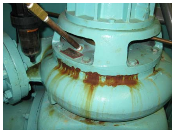
Terrace View Pumping Station, Rust on New Pumps
