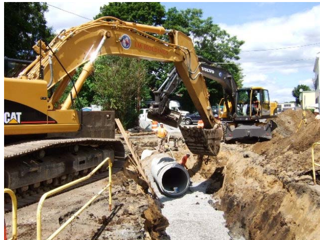
Figure 3. Example of open-cut pipe installation at Melrose, MA
