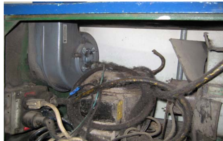
D Street NE Pumping Station, Hazardous Wiring
