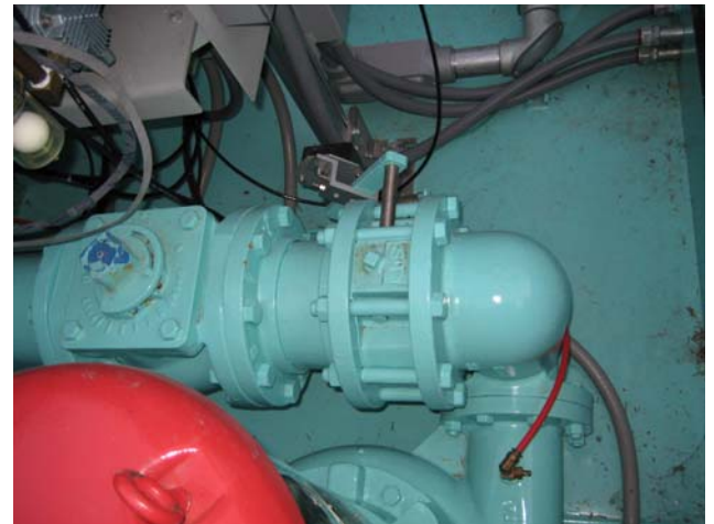
White Mountain Trails Pump Station, Custom-made Shot Radius Elbows that Plug
