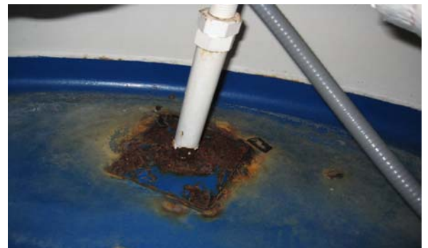
22 nd Street NE Pumping Station, Damage from Corrosion
