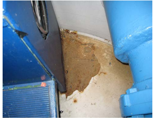
D Street NE Pumping Station, Floor Coating is Spalling
