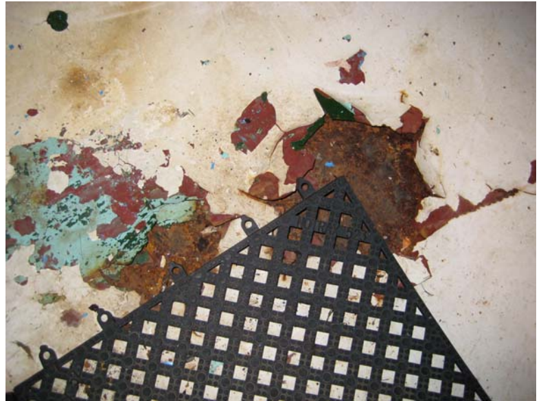
Ellingson Road Pumping Station, Corrosion of Floor
