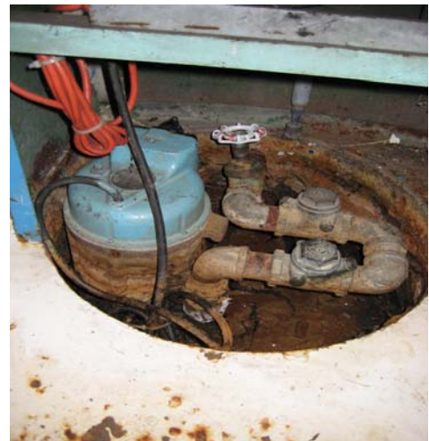
Ellingson Road Pumping Station, Corrosion in Sump
