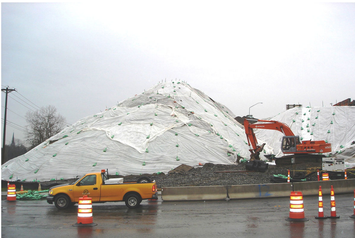
Figure IV-4-12. Material Covered with Plastic Sheeting
