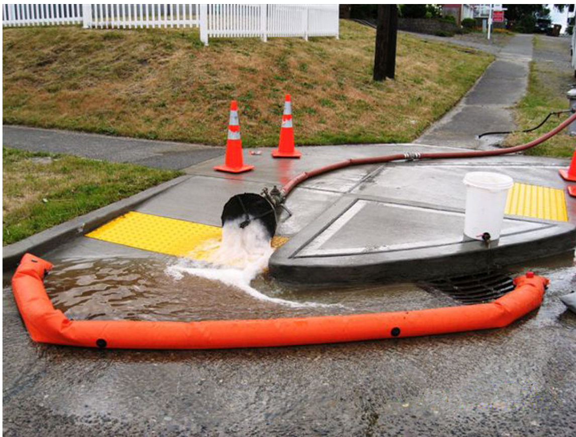
Figure IV-4-18. Hydrant Flushing
