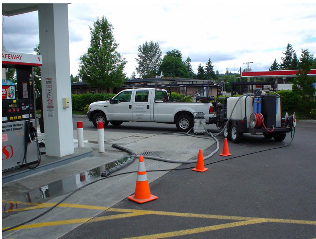
Figure IV-4-1. Pressure Wash Water Recovery System
