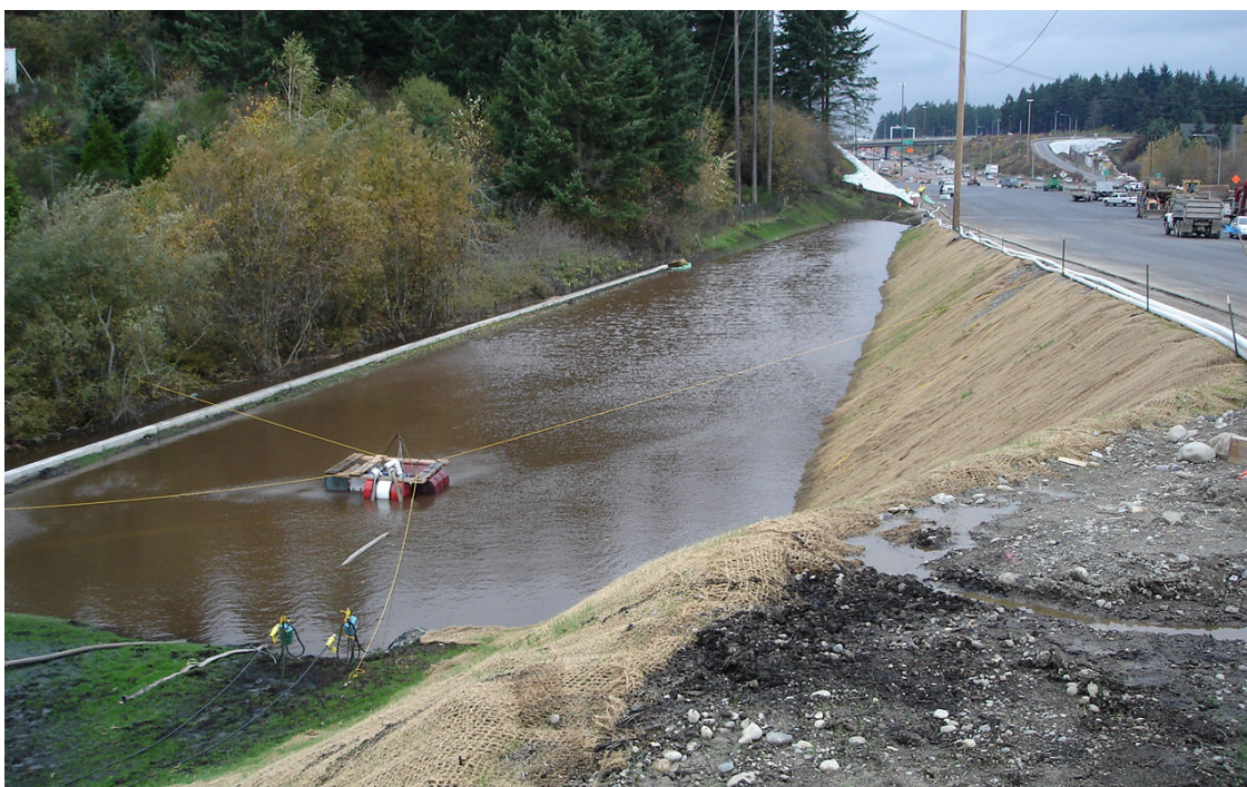
Figure II-3-37. Floating Platform with Struts
