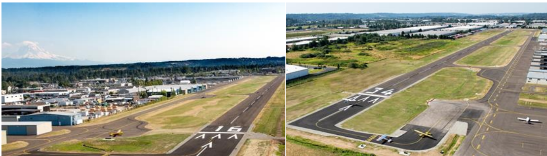
The Runway Enhancement project was completed in 2020, extending the length of runway 16/34 for increased safety and utilization.
