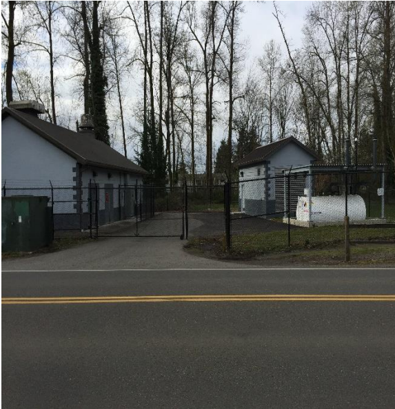
Green River Pump Station Emergency Power Station.
