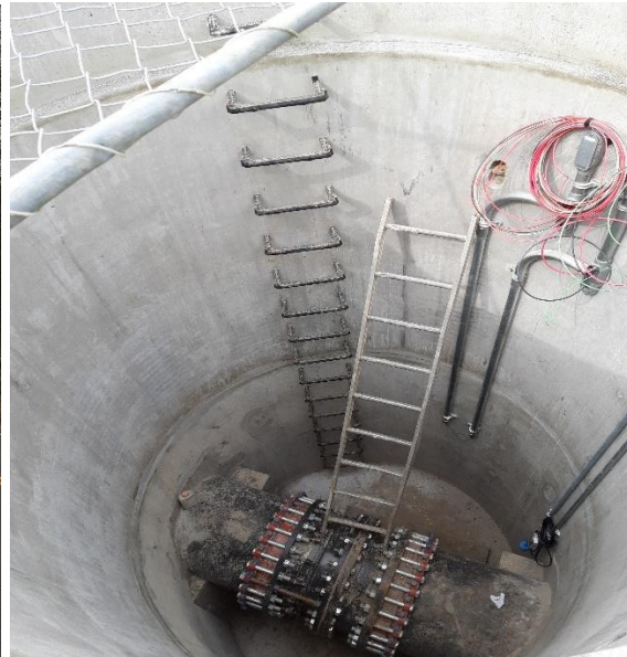
Reservoir 1 Seismic Control Valve project
