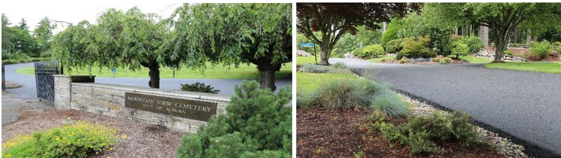
Completion of the repair and overlay of Cemetery Roads project in 2020.
