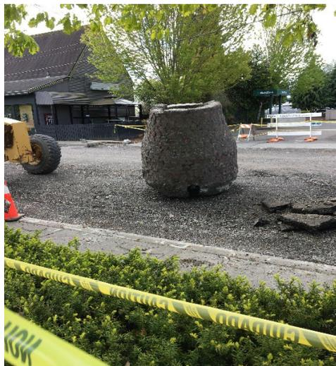
Brick sewer manhole replaced as part of the 2<sup>nd</sup> Street SE Preservation project
