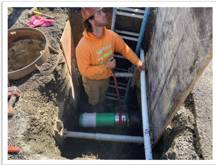
Spot repair on sewer main.
