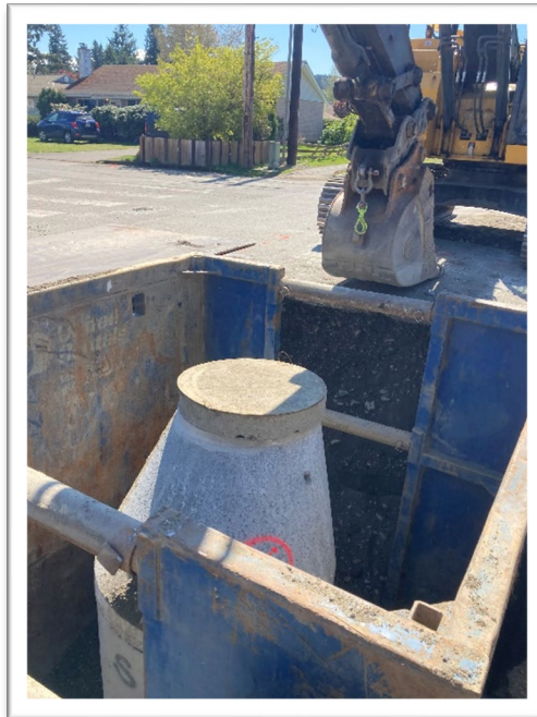
F St SE from 26 th to 27 th storm improvements.
