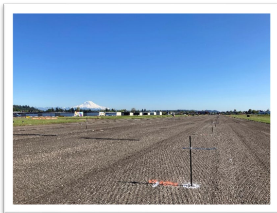
Airport Runway & taxiway rehabilitation project.
