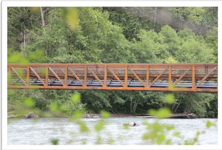
Coal Creek Springs 24-inch Transmission Main
