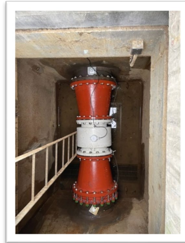
Coal Creek Springs Flowmeters Rehabilitation
