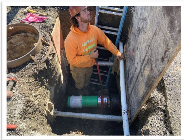
Spot repair on sewer main.
