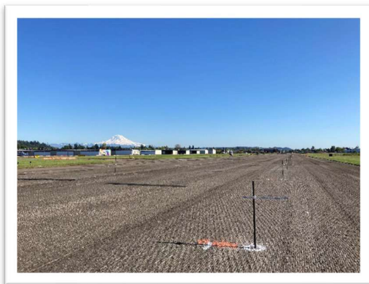
Airport Runway & taxiway rehabilitation project.
