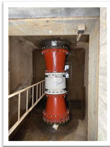
Coal Creek Springs Flowmeters Rehabilitation
