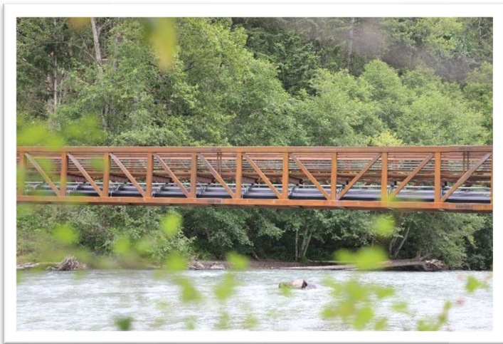
Coal Creek Springs 24-inch Transmission Main
