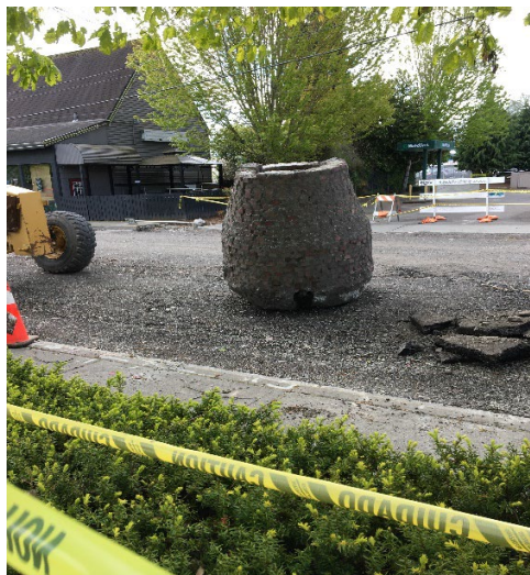
Brick sewer manhole replaced as part of the 2 nd Street SE Preservation project
