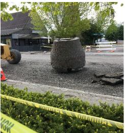
Brick sewer manhole replaced as part of the 2<sup>nd</sup> Street SE Preservation project
