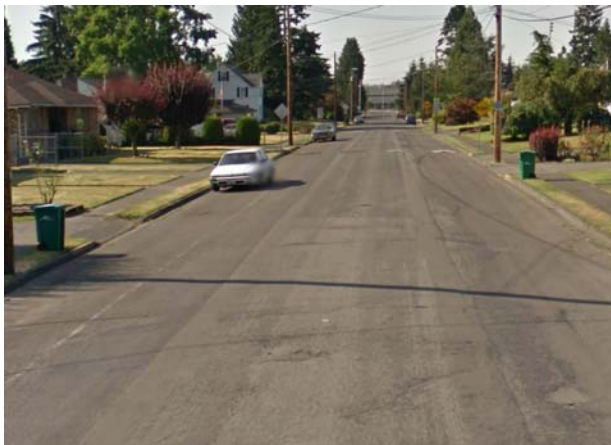
H St NE Before Rebuild
