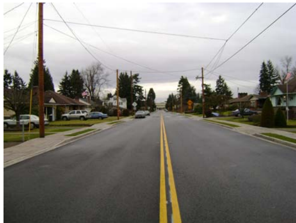
H St NE After Rebuild
