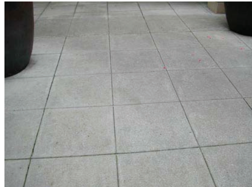
2'x 2' Scored Concrete with Light Brush Finish
